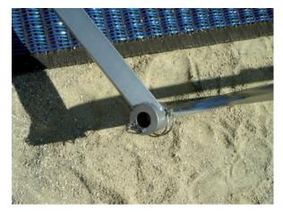
8. Installation of the starting straps with X connector (Mobi-Ma<sup>1®</sup> to Mobi-roll 'N Stow main shaft)
